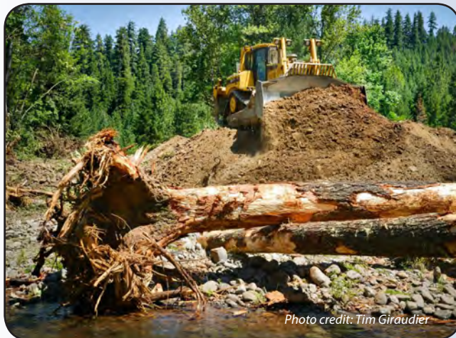
Berm removal and large wood placement underway at Staley Creek in 2017
